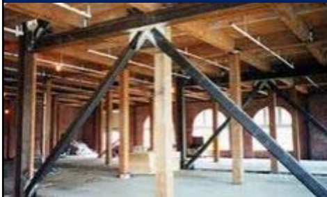
Interior cross bracing helps prevent building collapse
